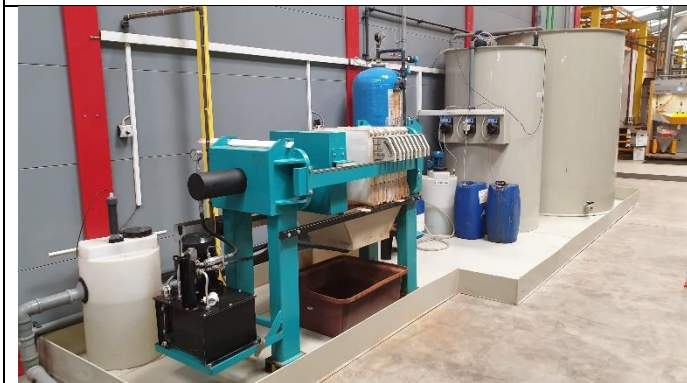
Fig. 3: Wastewater treatment plant, certified 0% environmental pollution impact
